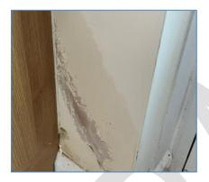
Picture 1: Rising damp to side of kitchen unit on external wall.
